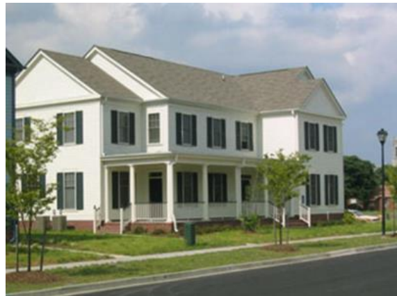
Figure C: Illustrative example of a small multi-family dwelling that resembles a large single-family dwelling.
