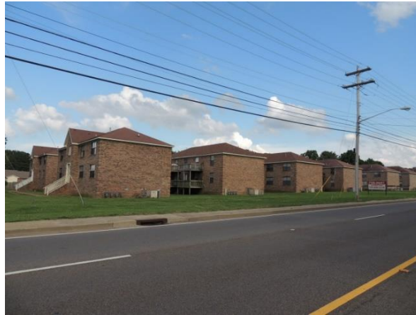
Figure B: Illustrative example of unacceptable architectural design for multi-family dwellings
